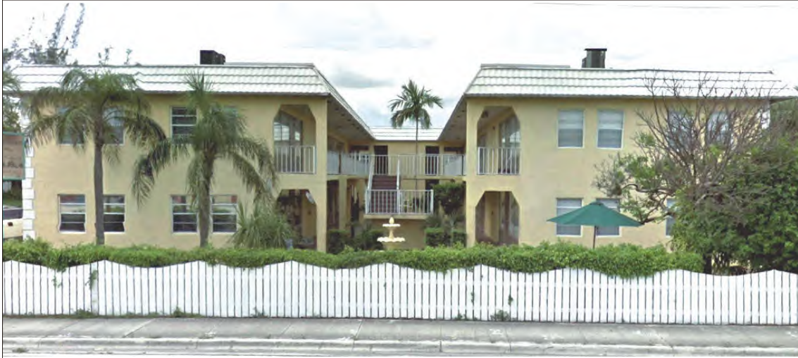
Figure 14: Thirty-Two Unit Multifamily Building Once Occupied by a Recovery Community in Oakland Park
